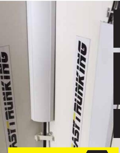
FIX BRACKETS OVER CABLES IN CORNERS OR ON FLAT SURFACES
